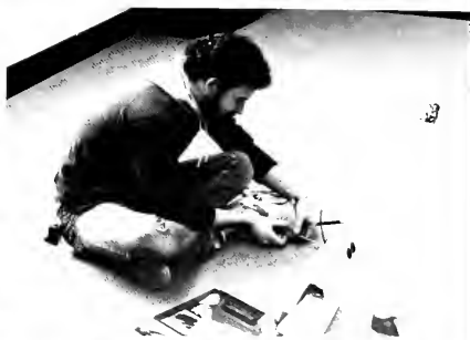
This construction worker puts the final touches on Jordan Hall renovations.
